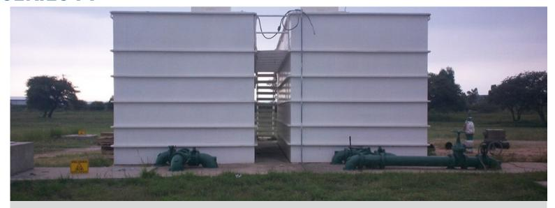
The Series 79 is designed to combine the processes of flocculation, settling, and filtration into a single tank, with flow rates ranging from 20 to 2,000 gallons per minute.
